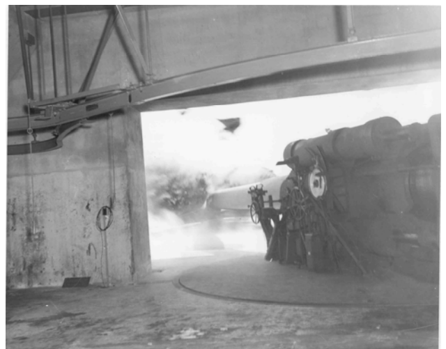
Battery Kingman - 2x12-inch Long Range Guns in casemate firing 1943
