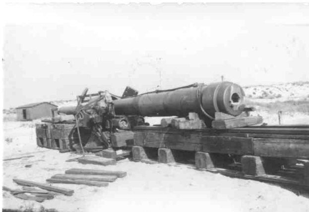
Assembling 6-inch M1900 rifle
