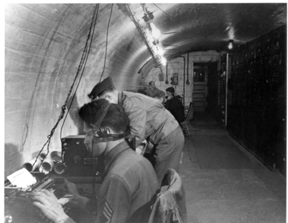
Switchboard Room, HDCEP, Ft. Hancock
