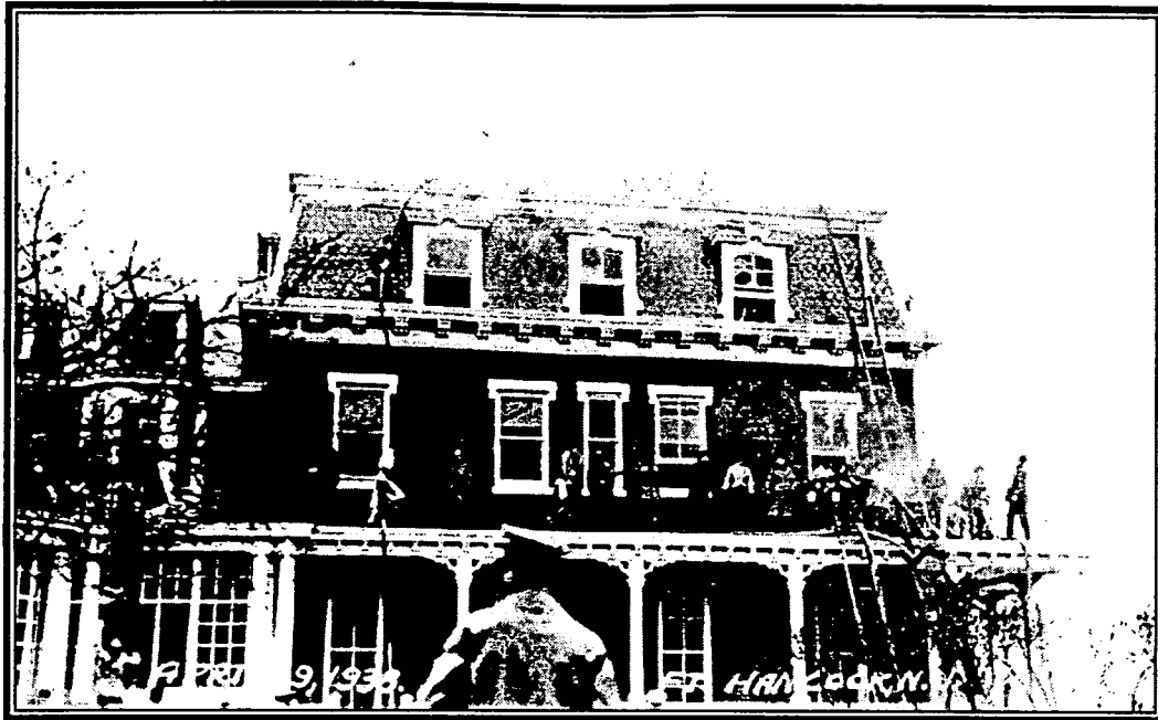
Figure 22: The Officers' Club (Brick House) at the time of the fire, April 1938, view looking north. The bay window and columns of the new dining room can be seen on the left. Photo from files (#2037) at Sandy Hook, Gateway NRA.
