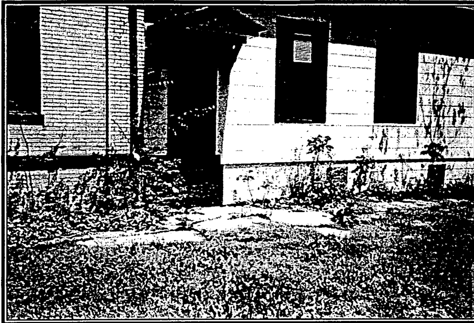
Figure 52: South facade of Officers' Club with concrete paving at doorway. Photo by author, 1998.
