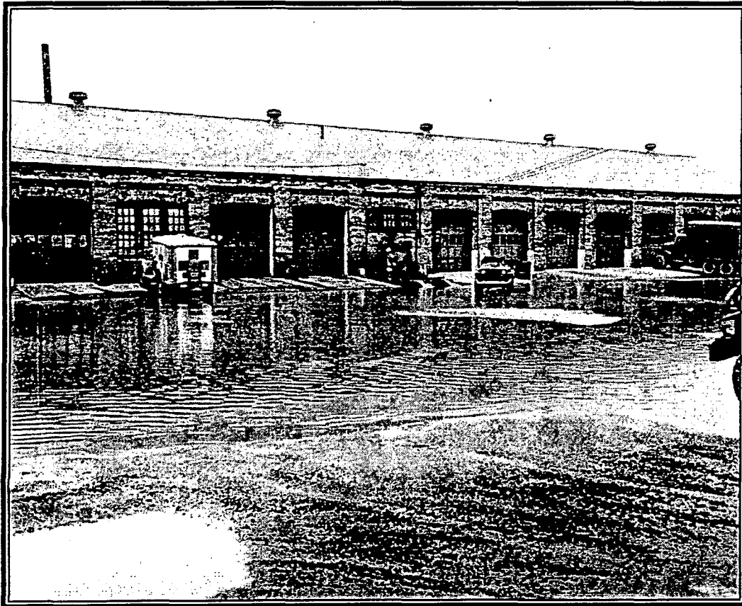
Figure 26: Maintenance area, Paint Shop, Building 132, c. 1945. Photo from Lent Collection (1945-111) at Sandy Hook, Gateway NRA.
