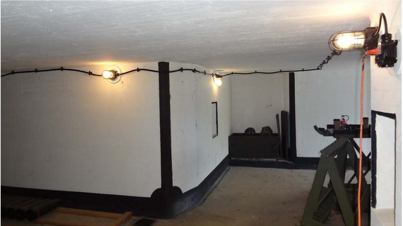
The view below shows the completed lighting inside the powder passage. Only a few cable hangers remain to be restored and installed. This is the lighting installation much as it looked from the late 1910s to the 1940s. The large racks on the right side of the wall are for gun implements such as ram-rods and cleaning staffs.
