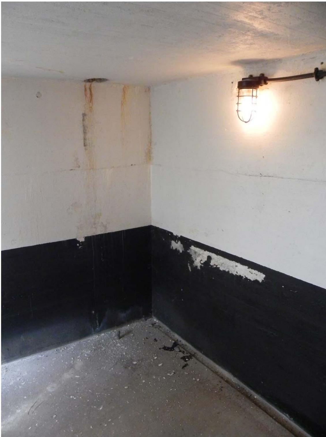
The photo below shows the results of running a paint knife across the wall...the paint just flaked off.
