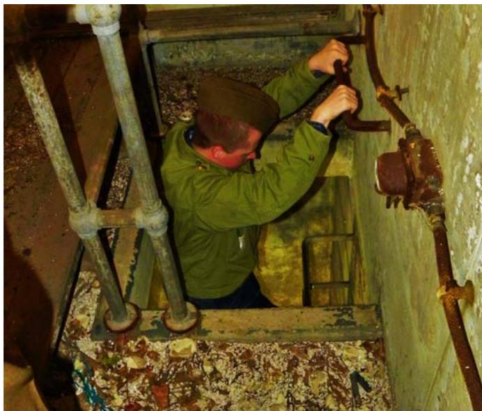
A detailed view of the interior is shown here. Note the different heights of the pedestals (right, and center). The different heights (and corresponding observation slits) allowed two separate azimuth instruments to be used simultaneously.
