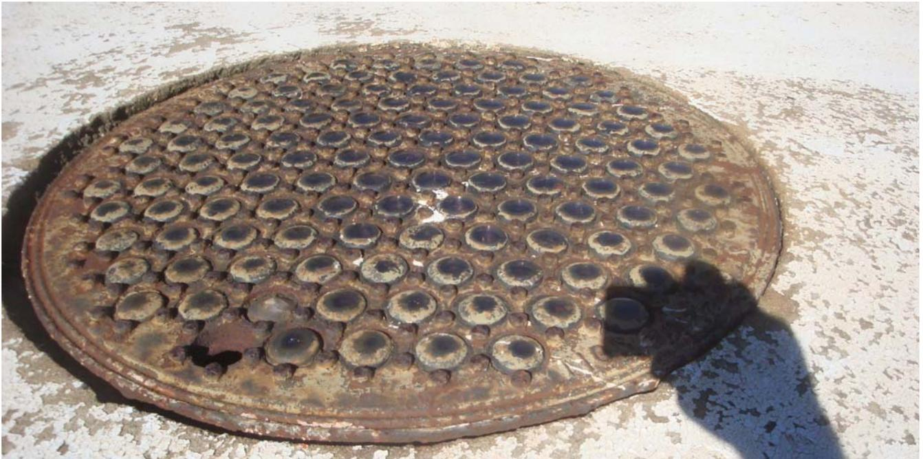
The photo below shows the glass light inserts from the inside of the cable hut. This is a unique and effective way to provide lighting inside the cable hut to enable the Signal Corps personnel to work on the telephone wires without requiring additional lighting.
