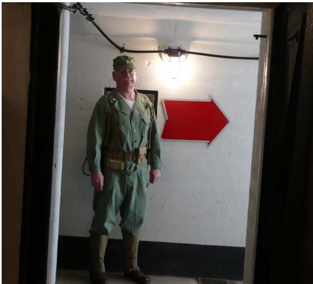
A second 1915 standard COE wall light was installed in the entrance to Gun #1 shell hoist and magazine. The Gun No. 1 side (or right-hand side) of the Shell and Powder Magazines, as well as the Powder Passage, have been exclusively rewired not only with these original fixtures, but with cables that have been run along original pathways and using original 1915-era US Army COE cable hangers.
