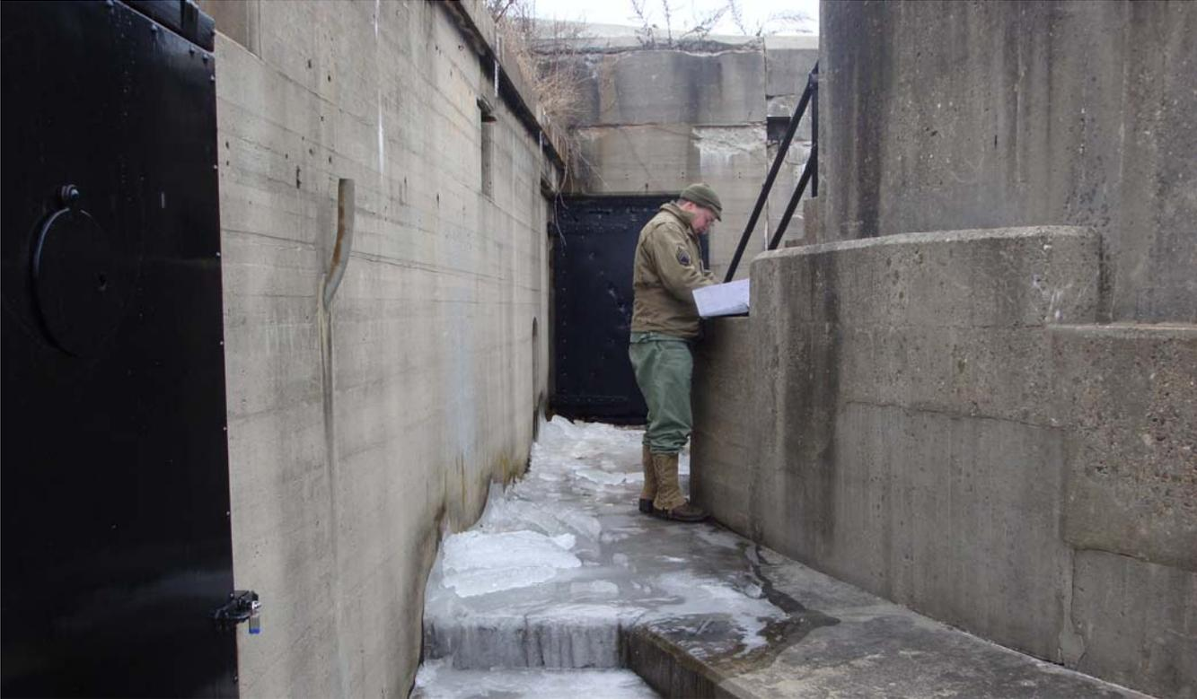
The amount of ice at the battery is apparent in the photo of SSG Weaver below. One of AGFA's goals is to refurbish the original concrete gutter drainage system at the battery, thereby preventing such dangerous overflows and buildups of ice on level surfaces.
