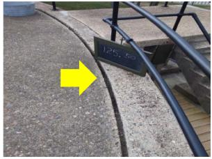
The photo below at the base of Gun #1shows the concrete patch on the small arc that has been applied in contrivention to the original drawings. This patching will be removed and replaced by expansion joint material. We have no idea who placed this patching material in this location. The original drawings make it clear it does not belong.
