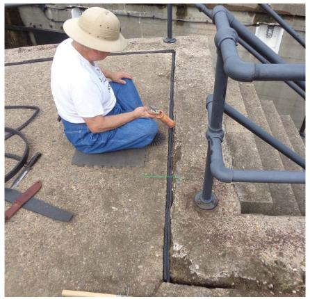
Removing the "patching cement" from the short arc next to the gun proved to be impossible by hand. The answer was a 1941 Black and Decker electric hammer shown below. This hammer was perfect for the job - just strong enough to remove targeted material without disturbing original concrete fabric.
