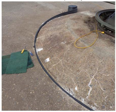
The photo below shows the expansion joint with full sealing treatment applied to about half of the short arc up to the drainage trough.
