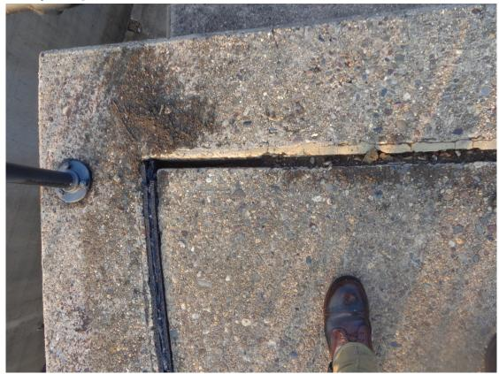
The photo below shows a wider view of the area above. Completed expansion joint is on the right. This was as far as the work proceeded on 27 August.
