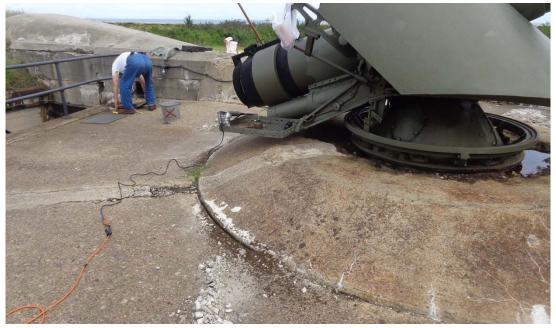
The final work was undertaken on 10 October. All that remained to be done was clean out all the remaining debris in the small are and install the expansion joint. The 1941 Black and Decker Electric Hammer proved perfect for this task. The photo on the left is during the work and the right after.
