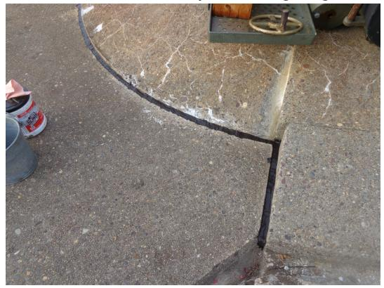
The photo below shows the end of the arc and the short run to the drainage trough fully installed and sealed with KoolSeal asphaltic sealer.
