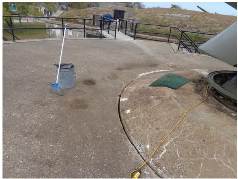
The photo below shows the small arc and short run to the drainage trough completely cleaned out and ready for expansion joint.
