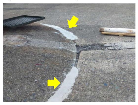
AGFA recommended installing quarter inch expansion joint (layered) to fill the expansion crack. This area is between a half inch to one and a half inch wide. We recommend roll expansion joint in half inch thicknesses. The expansion joint material will be placed in double and triple thicknesses based on width of the joint, joined with black sealer and cold asphaltic sealer.
