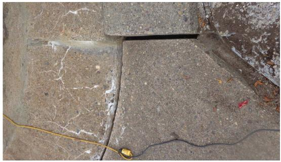
The photo below shows the installation of two strips of expansion joint around the small arc. The removal of debris was quite effective and it was deep enough to enable the entire run of expansion joint to be 4-inches deep.
