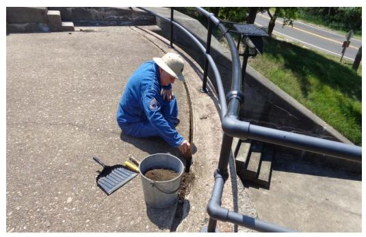
The photo below shows the work done by TSG Weaver to clean out the large arc. However, a number of jammed stones resulted in some portions of the expansion joint only being about 3 inches thick instead of four inches.
