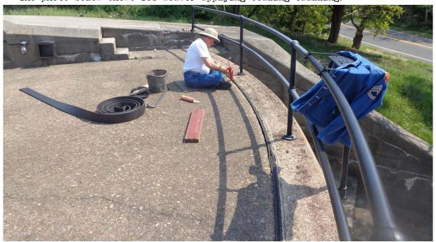
The photo below shows the large arc terminating point with expansion joint in place prepared for sealing. The horizontal expansion trough (top of powder passage stairs) is still filled with dirt and debris that must be removed prior to joint placement.
