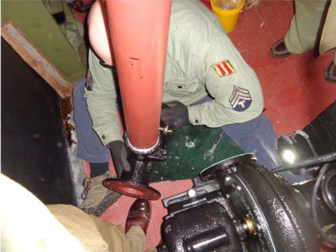
Below the team continues to seat the lower valve and the bypass pipe.
