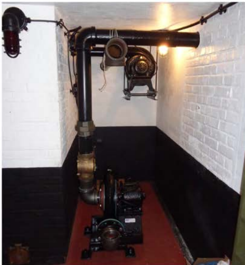
The photo below shows the motor and blower proper.
